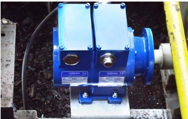
After: Electronic position switch ERC 40 replaces mechanical cam limit switches.
