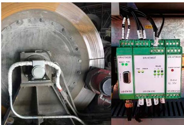
After: Hoist drum with U-ONE basic unit and holding brake. The photo right shows the U-ONE electronic modules in the switchboard.
